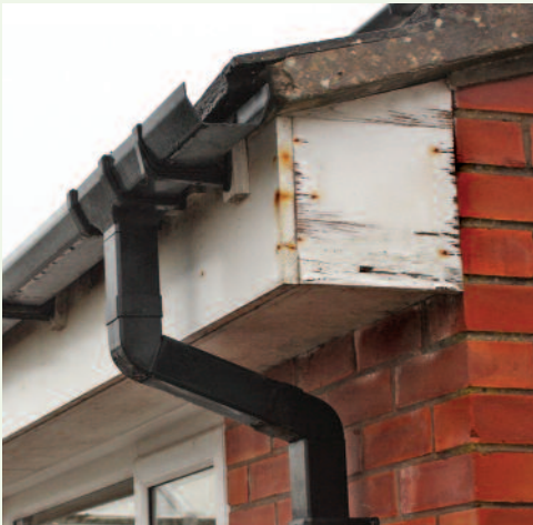
Timber roofline can rot without maintenance...
