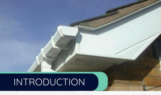
Bargeboards are an essential architectural element typically found on the gable ends of a property, which is the triangular portion of a wall between the edges of a sloping roof. The box ends, also known as bargeboard ends, are the decorative or functional elements at the extremities of these bargeboards.
